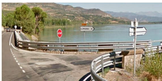
Control 5 Pont Cellers
